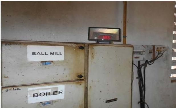
Fig - 3: POKA-YOKE on temperature panel.
