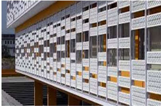
Figure:12 Facade with Jali
