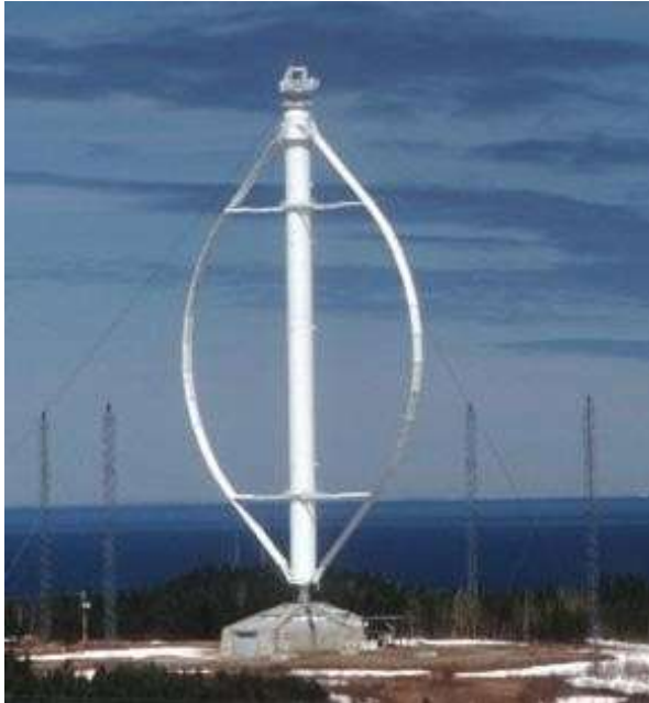
Fig 1. Eole C, a 4200-kW vertical axis Darrieus wind turbine with 100 m rotor diameter at Cap Chat, Québec, Canada. The machine, which is the world's largest wind turbine, is no longer operational. Danish Wind Turbine Manufacturers Association.
