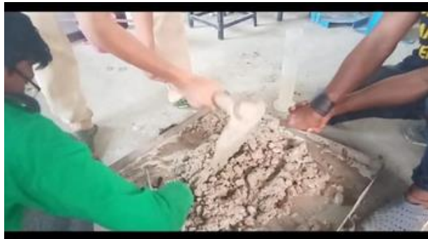
Fig.7 Dry and Wet Mixing of Concrete
