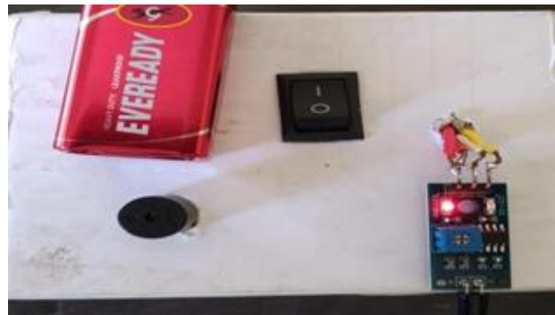
Figure 2: Fire Alarm System
